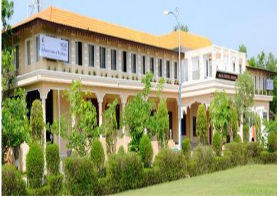
Auditorium with 1200 capacity
