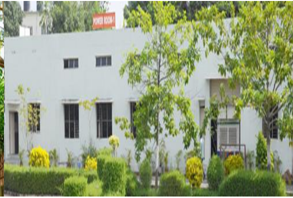
Power Backup Rooms
