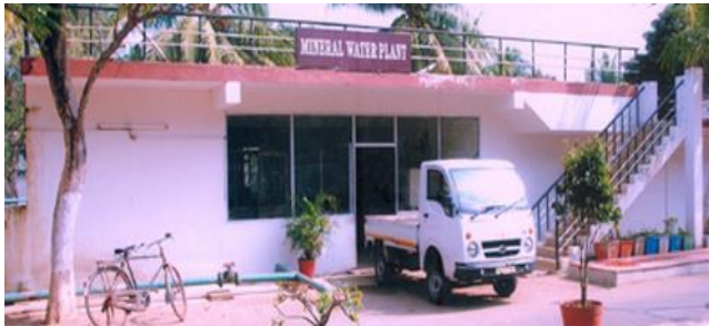
Mineral Water Plant
